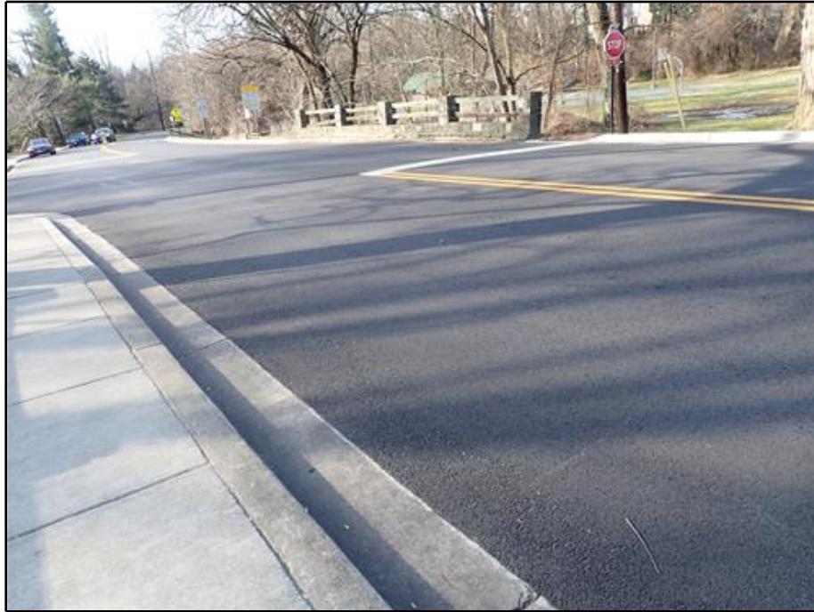
7. General View of Roadway over Structure (Looking South)
