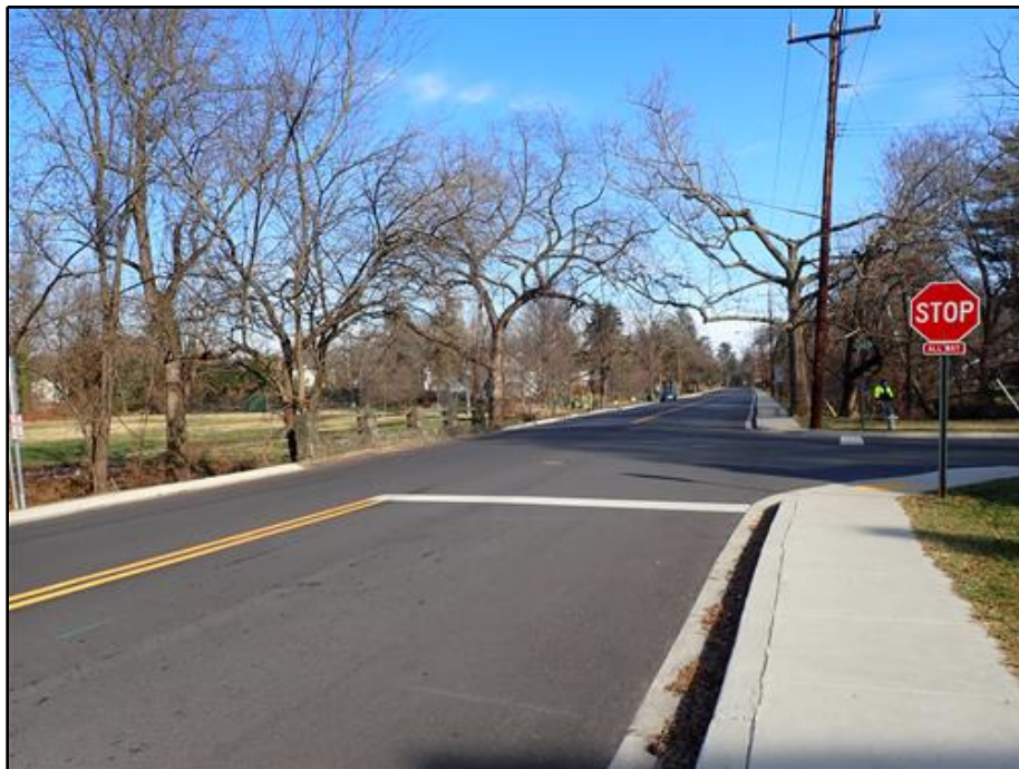
2. South Approach Looking North
