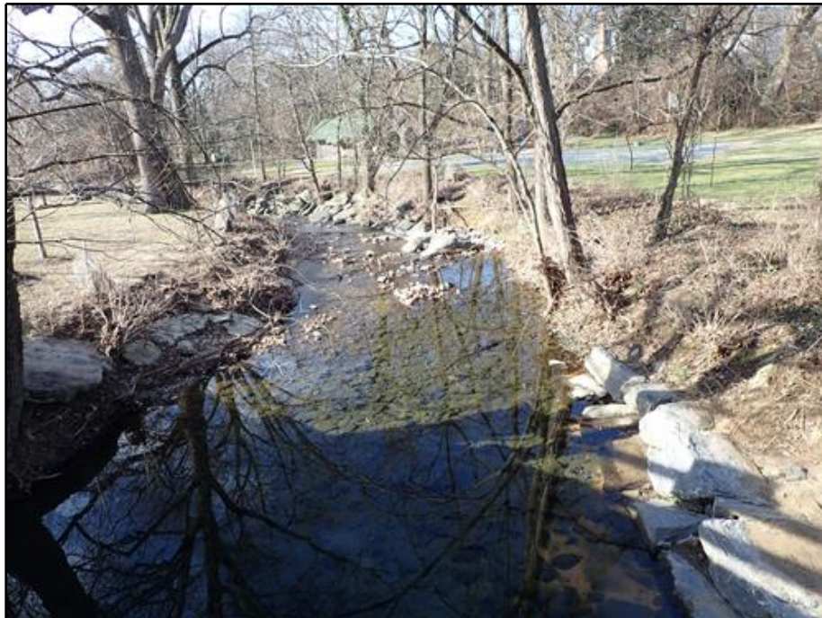
6. Looking West (Downstream)
