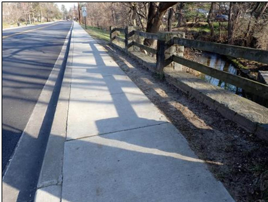
8. East Sidewalk (Looking North)
