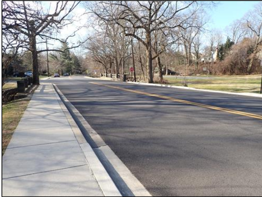
1. North Approach Looking South
