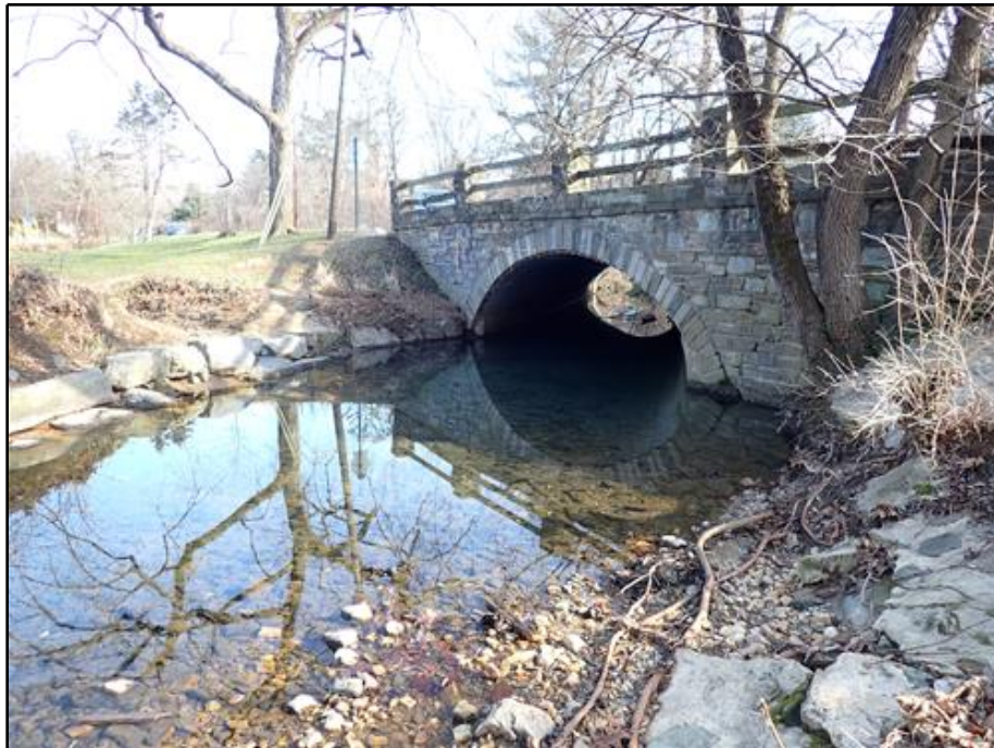
4. West Elevation (Downstream)
