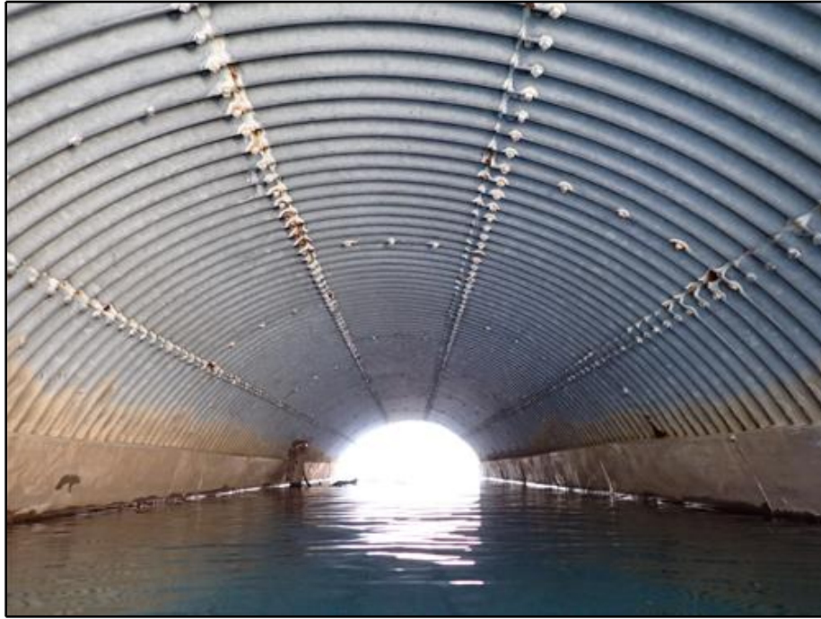
9. Typical Arch Underside (Looking West)
